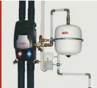
Installation of hydraulic unit for connection of ground-to-brine heat exchanger system
