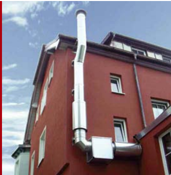
Outdoor installation with wall bracket (accessories).
