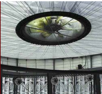
"Balancing act" at EXPO in Hannover. One main fan with \varnothing 2800 mm and as well as 40 further fans, arranged in a spiral shaped have been used to achieve the biggest artificial tornado in the world with a height of 22 m.
